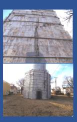
This base is octagonal shaped with each side being approximately 10 feet wide and 20 feet high. In the 1950's the concrete base was wrapped with five (5) steel bands to help stop the shifting that was being seen.
