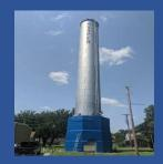
The 125-foot tall and 135,000-gallon standpipe was constructed in 1887 and has been in continuous operation since 1907. The original foundation base is limestone. In the early 1900's the limestone base was encased in concrete.
