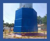
The carbon fiber is susceptible to UV light and if installed outside needs to be sealed to be protected.
