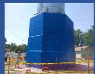
The carbon fiber is susceptible to UV light and if installed outside needs to be sealed to be protected.
