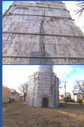
This base is octagonal shaped with each side being approximately 10 feet wide and 20 feet high. In the 1950's the concrete base was wrapped with five (5) steel bands to help stop the shifting that was being seen.
