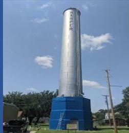
The 125-foot tall and 135,000-gallon standpipe was constructed in 1887 and has been in continuous operation since 1907. The original foundation base is limestone. In the early 1900's the limestone base was encased in concrete.
